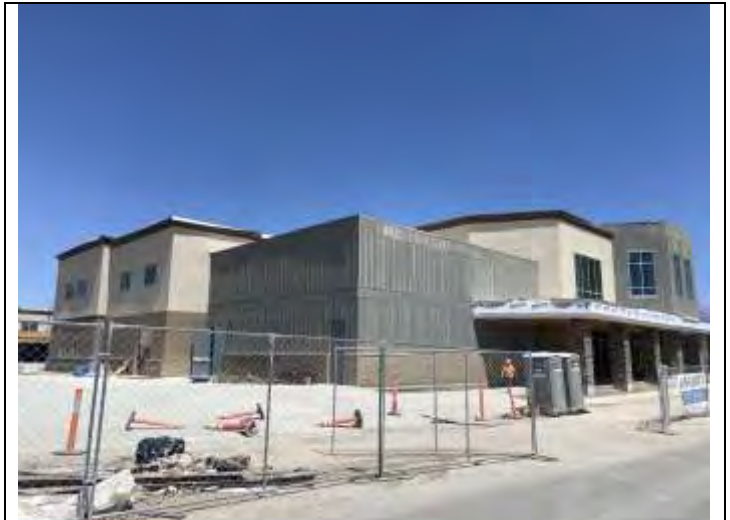
20. Exterior finishes of the subject building.
