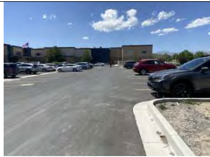
15. General grounds – asphalt paving.
