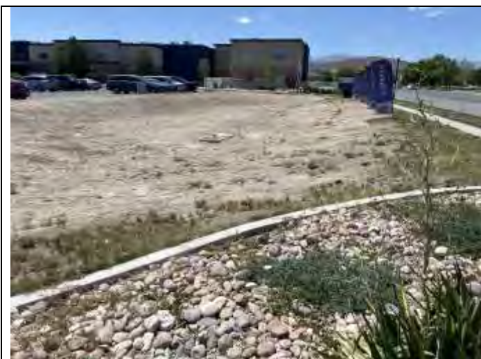
59. Storm water detention area.
