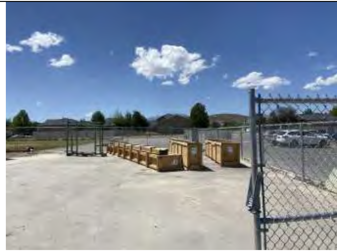
17. General grounds – southern section of the property.
