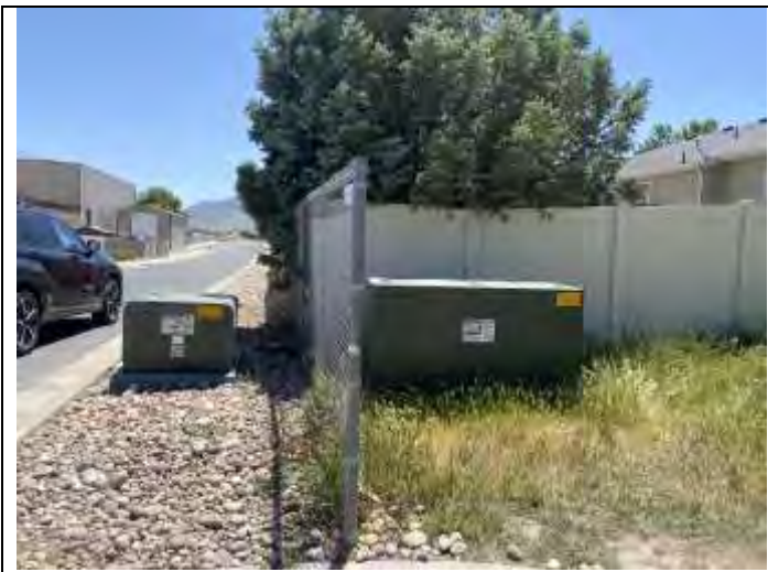
5. West perimeter of the subject property, looking north.
