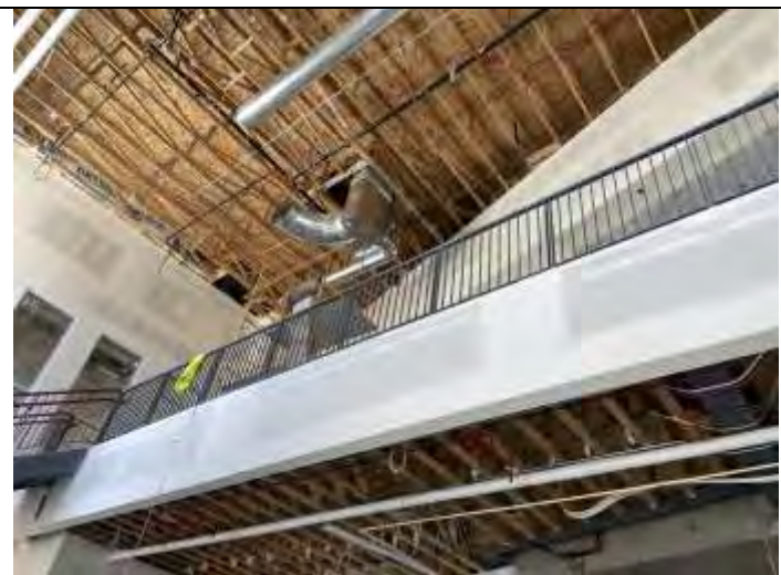
40. Construction in progress.
