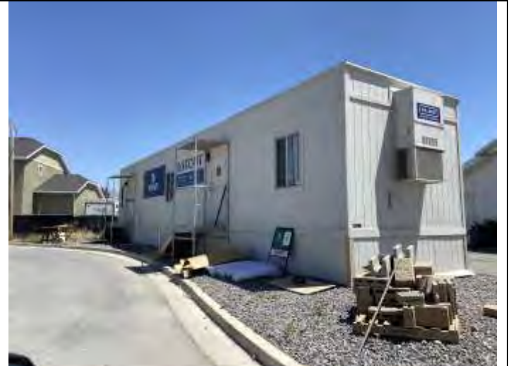
14. General grounds – construction trailer.
