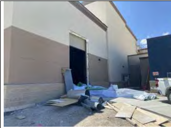
21. Exterior finishes of the subject building.
