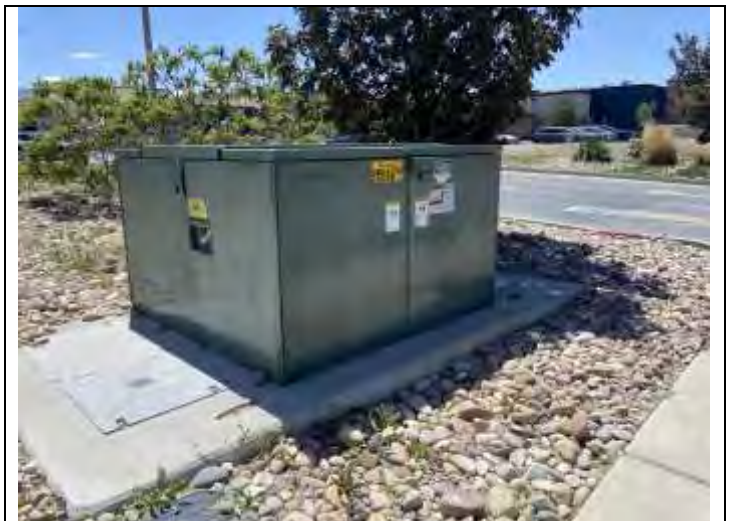
44. Pad-mounted transformer.
