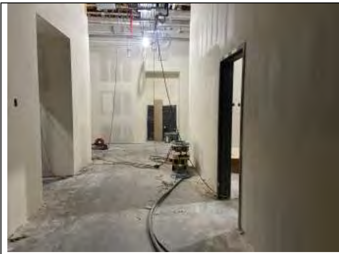
37. Construction in progress.
