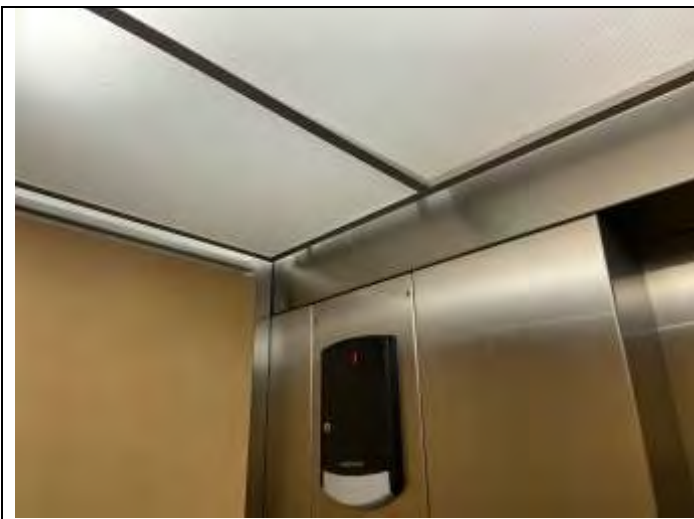
47. Elevator cab finishers.
