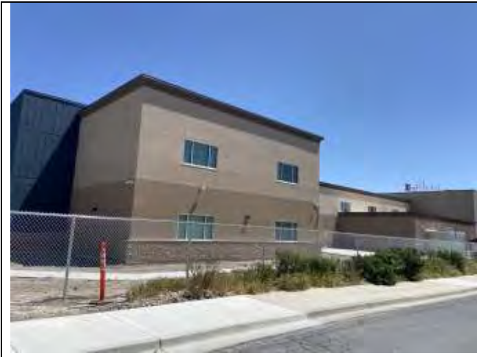
19. Exterior finishes of the subject building.
