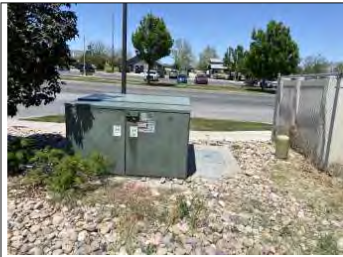
43. Pad-mounted transformer.
