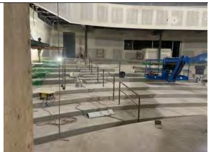
36. Construction in progress.
