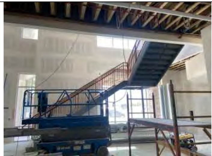
38. Construction in progress.
