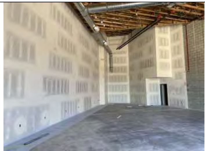
34. Construction in progress.
