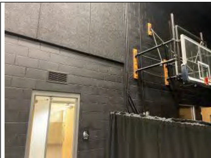
23. Interior finishes of the subject building – gym.
