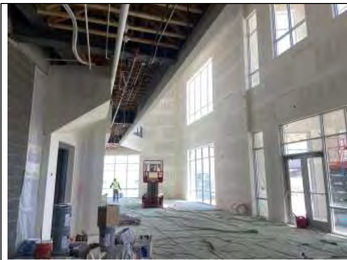
39. Construction in progress.
