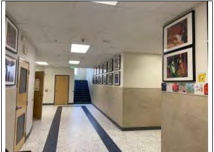
22. Interior finishes of the subject building – hallway.
